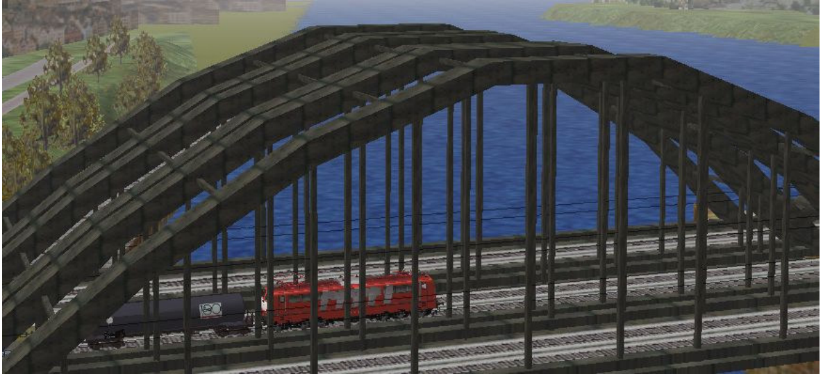
One of the spans of the six-track Hohenzollen Bridge Köln
